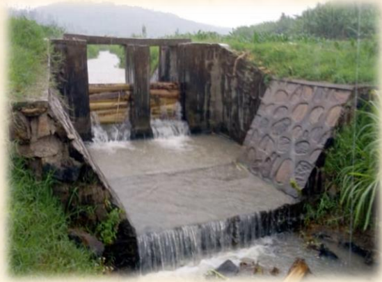
PHOTO 10: POOR QUALITY OF IRRIGATION WATER DUE TO EROSION AND REPARATION USING BANANA STEMS DUE TO DAMAGED DOORS.
