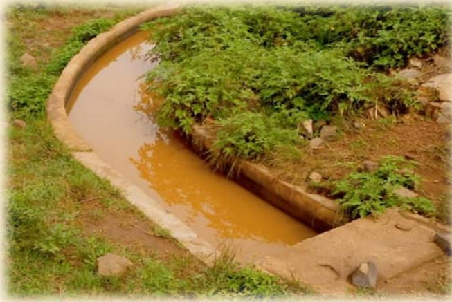
PHOTO 10: POOR QUALITY OF IRRIGATION WATER DUE TO EROSION AND REPARATION USING BANANA STEMS DUE TO DAMAGED DOORS.
