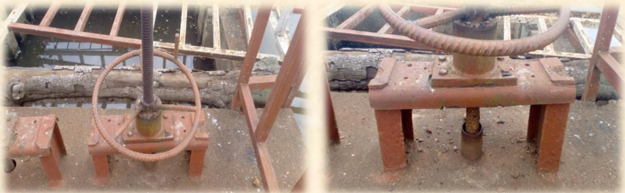
PHOTO 7: NONFUNCTIONING WATER CONTROL VANE IN THE CYUNUZI IRRIGATION SCHEME
