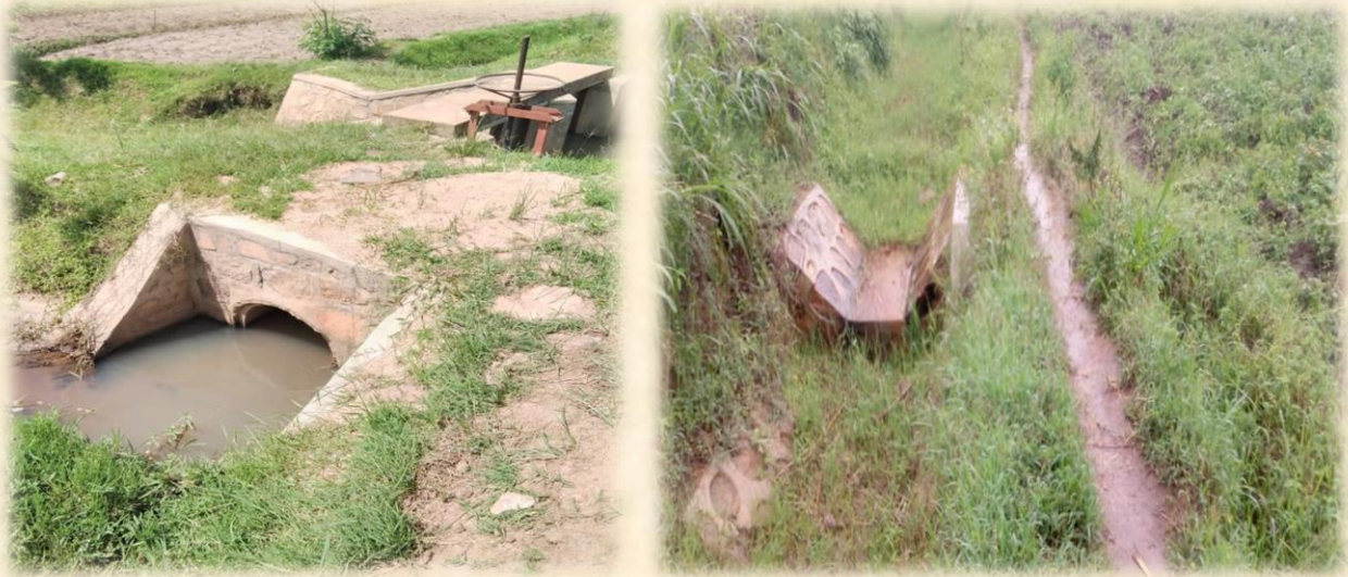
PHOTO 4: CURRENT STATE OF KIBUZA AND RUBOROGA IRRIGATION SCHEME CHANNELS IN KAMONYI 18
